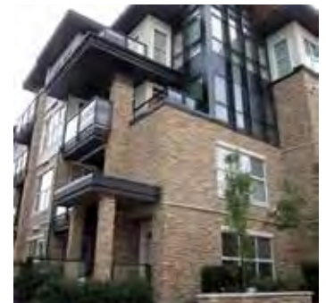
Outdoor Terraces Raised Above Street Grade
