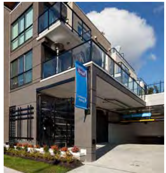
Garbage and Recycling Enclosed within a Building
