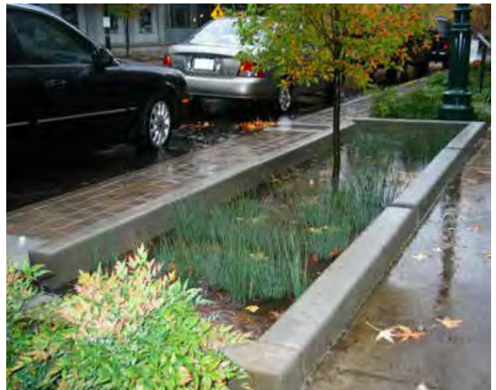
Rain Garden Collecting Run Off from Road and Sidewalk
