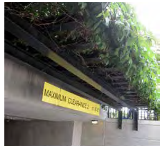
Trellis Over Parkade Entrance
