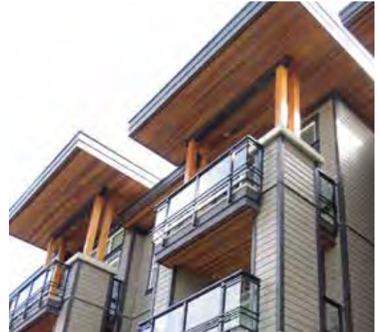
Cedar Soffits Protected from Weather
