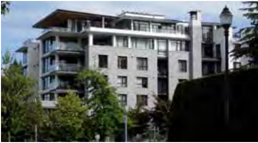
Upper Storey Set Back to Reduce the Building's Impact
