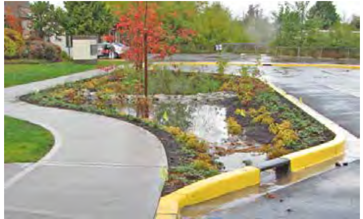
City of Tacoma's Rain Garden Bump Out
