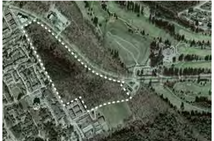
Aerial View of Existing Site
