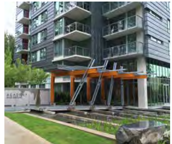
Highrise with Strong Entry Utilizing Water and Real Wood
