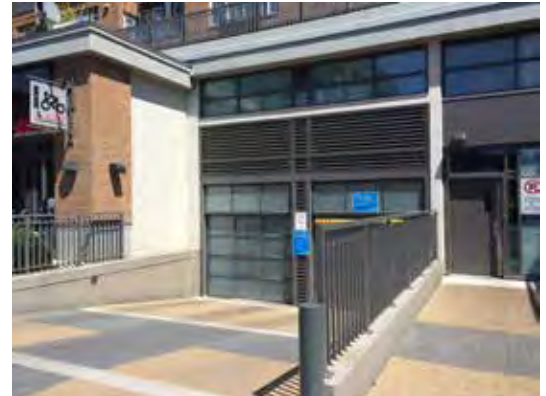
Loading Bay with Doors
