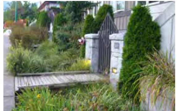
Boardwalk Crossing Over Bioswale
