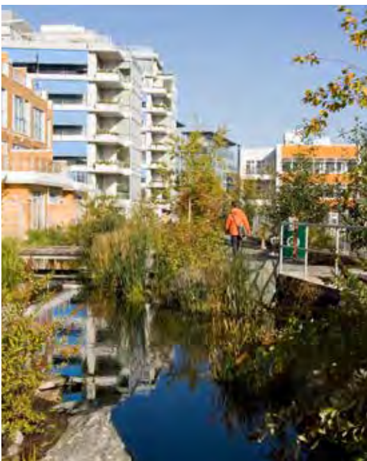
Dockside Green Development Residential Frontage on Stormwater Management System
